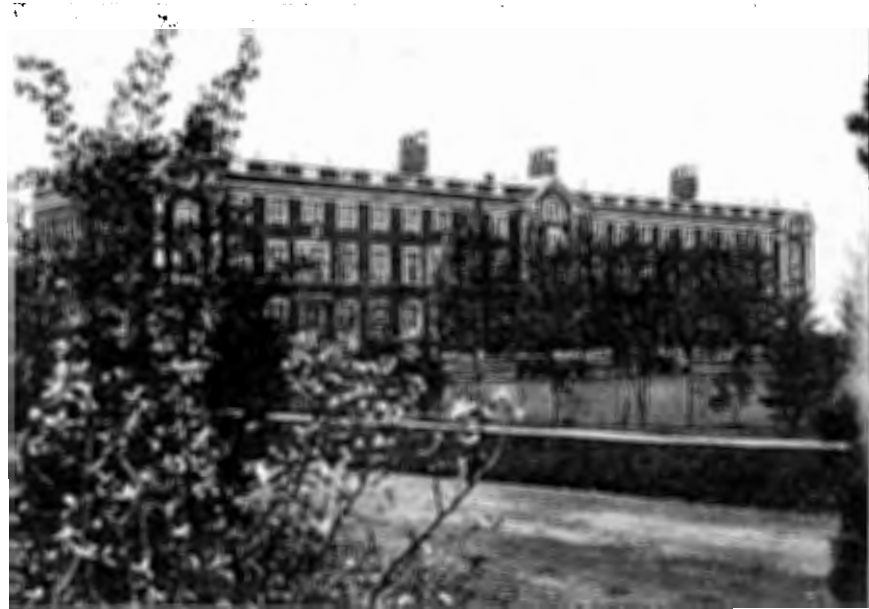
ARTS BUILDING, UNIVERSITY OF ALBERTA
